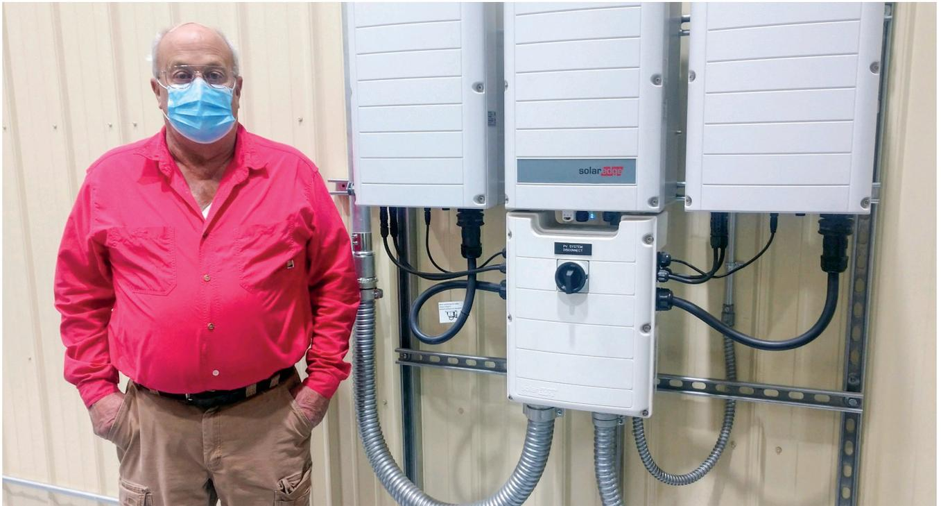
Highway 83 Lawn & Leisure owner **Russell Gohl** stands next to the solar control panel regulating the solar energy coming into the building from its 300 roof-mounted solar panels.
